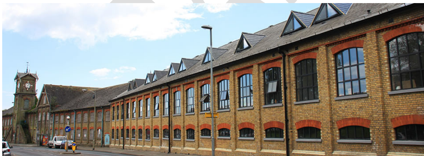
Buckland Mill Development
